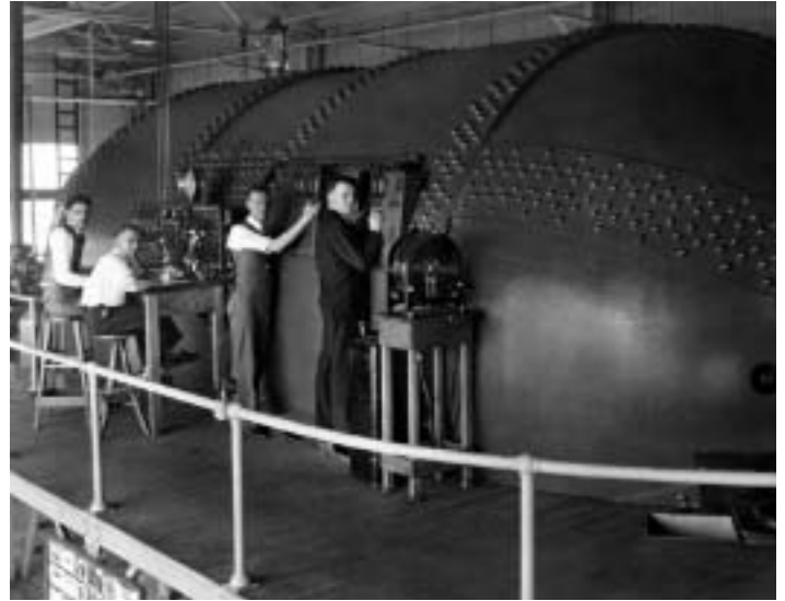
In this photo taken on March 15, 1929, NACA staff members conduct tests on airfoils in the Variable Density Tunnel. In 1985, the Variable Density Tunnel was declared a National Historic Landmark.
