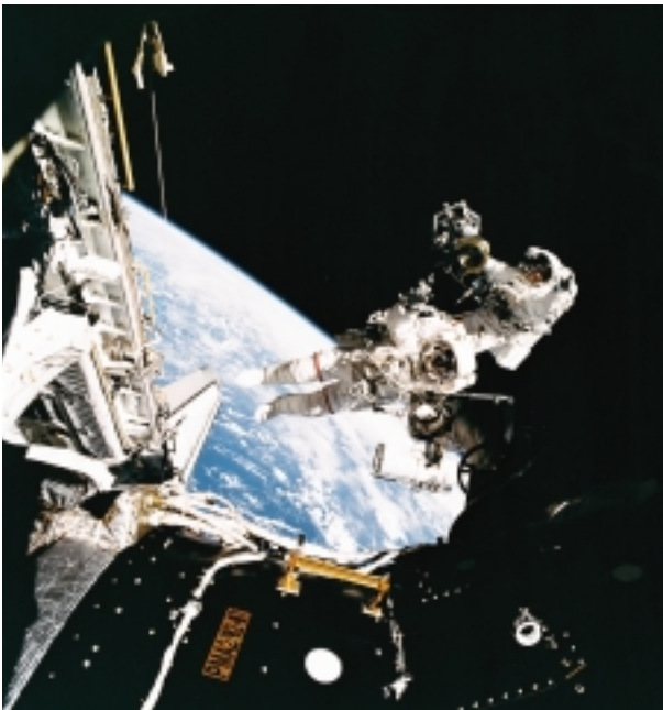
NASA astronauts work to attach a Russian crane to the International Space Station in preparation of future assembly.
