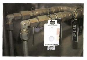
to be exposed and observed. In the presence of either hydrazine or MMH, both tapes change colors, providing an immediate visual alarm.
