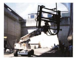
The decoating system can reach high surfaces, eliminating the need for scaffolding.
