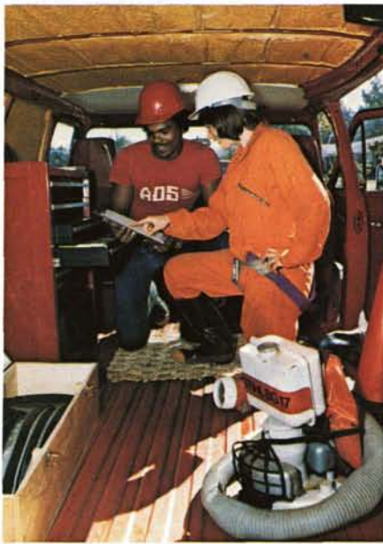
An American Digital Systems field crew prepares to install a sewer waterflow monitoring system. The system, an aerospace technology spinoff, is shown in the foreground.
