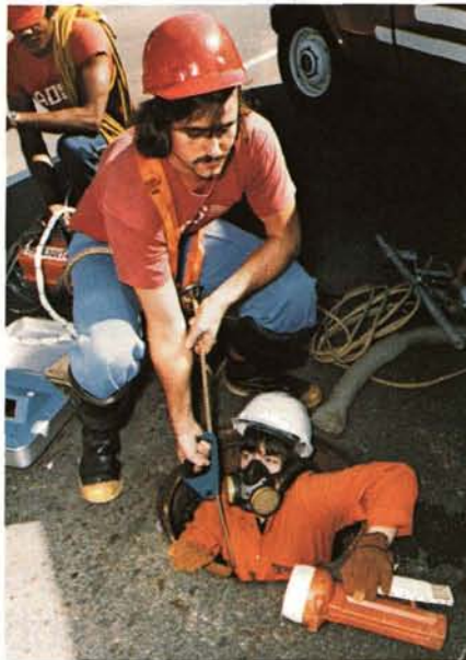
While one technician mans a safety line, another descends into a sewer to position the waterflow monitoring equipment. The system helps locate pollution-causing sewer leaks.
