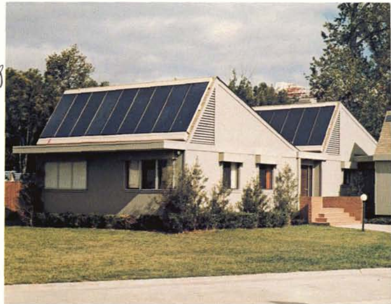
Tech House, located at NASA's Langley Research Center, Hampton, Virginia, is a demonstration project in which aerospace and commercial building technology are combined to produce an energy-efficient home. Advanced technology offers savings to the family in utility costs and energy conservation.
