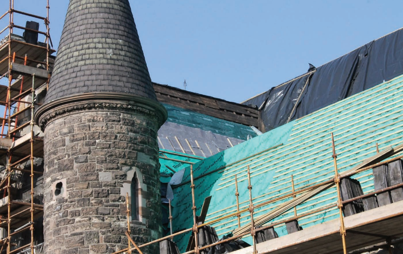
Insulation made with Aspen Aerogels' Spaceloft product is used to renovate a historic building in Belfast, Northern Ireland.
