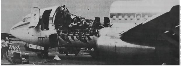
A photograph taken of Aloha Airlines Flight 243 in April 1983 after it made an emergency landing. Unexpected fatigue cracking led to the structural failure of the top half of the fuselage, exposing crew and passengers to the elements. NASA aeronautics engineers used cutting-edge software known as Structural Analysis of General Shells to help determine the cause of the incident.
