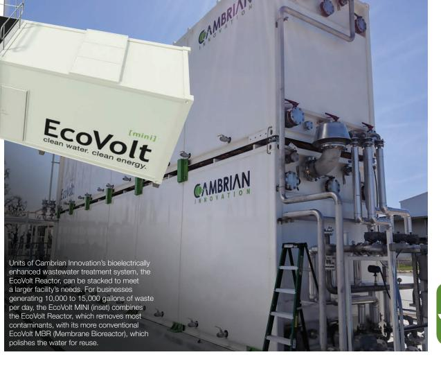
With the help of its living electrodes, the EcoVolt Reactor can reliably process more variable loads of wastewater than other anaerobic systems with minimal oversight, all while achieving high treatment and methane production rates, the company says.
