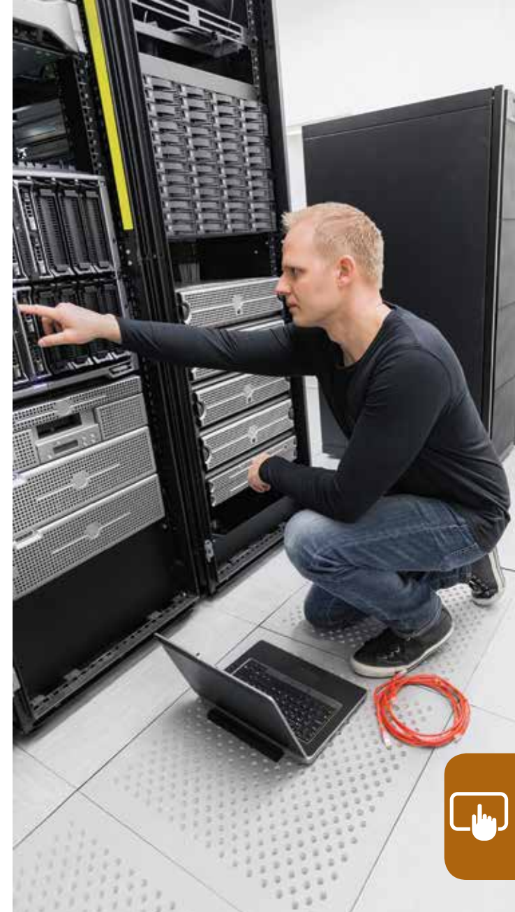
The Canonical Distribution manages and even automates many tasks that until now have required engineers to visit data centers.
