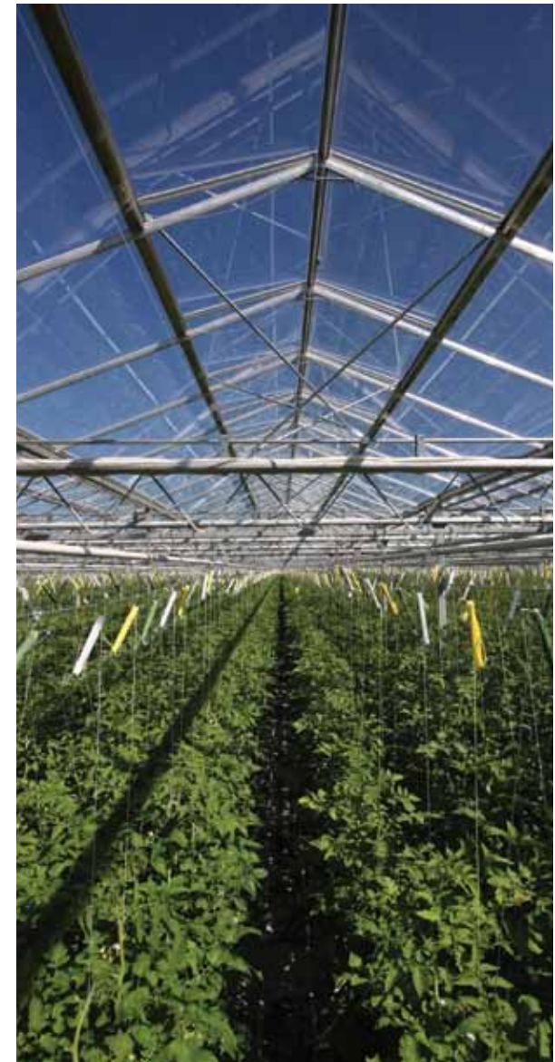
GreenField Solar's concentrators produce an excess of thermal heat that can be used for secondary purposes, such as heating nearby buildings or even greenhouses.
