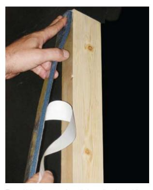
Thermablok strips are easily applied to wall studs, providing an affordable and environmentally friendly boost to a wall's insulation factor.
