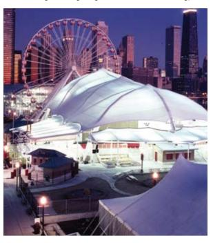
Apollo-era space suit fabric proved useful for designing visually intriguing, large-scale, permanent tensile fabric roofs, like the one seen here at Chicago's Navy Pier.
