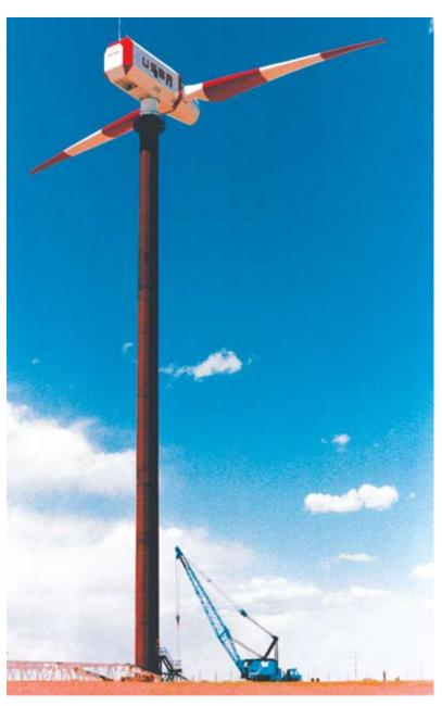
first multimegawatt wind turbine, was developed—capable of providing electricity to thousands of homes. Successive experimental models (13 in all) were built throughout the country. Viterna notes that these were also record setting in size and output; the 4-MW capability of the WTS-4 turbine, built in 1982 in Medicine Bow, Wyoming, was not surpassed for about 25 years.
